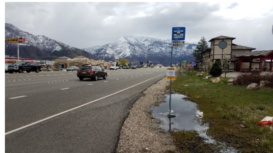
FIGURE 1 - NON-COMPLIANT UTA BUS STOP
